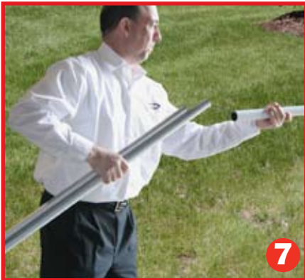
7 Remove each pole from the carry bag and carefully assemble them using the bungee cord as your guide. Once your pole lengths are together, make sure the hook eyelets are all facing the same direction and along the same line of site for an even flag installation.
