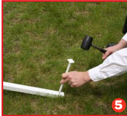
5 Remove the ground spikes from the leg storage and place the spikes through the holes on the end of each leg. Using the rubber mallet supplied, pound the spikes into the ground for a secure installation.
