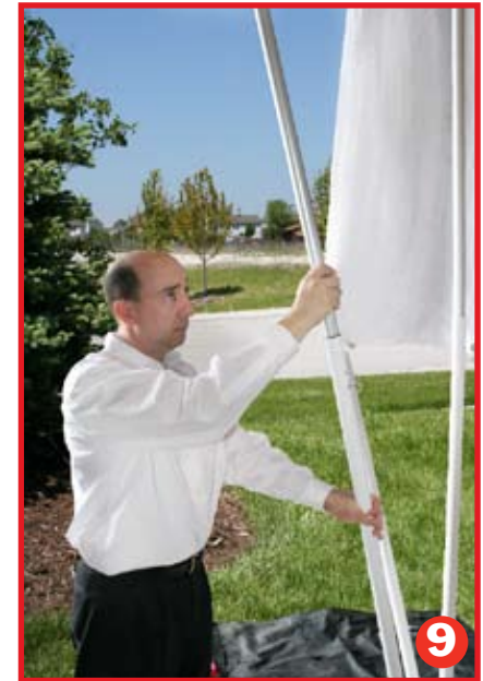
9 Carefully place each pole into the base in it's proper location. The center pole should go first followed by the surrounding poles. Try to balance each side of the base as you install the poles so you do not have all of the weight on any one side for any length of time.
